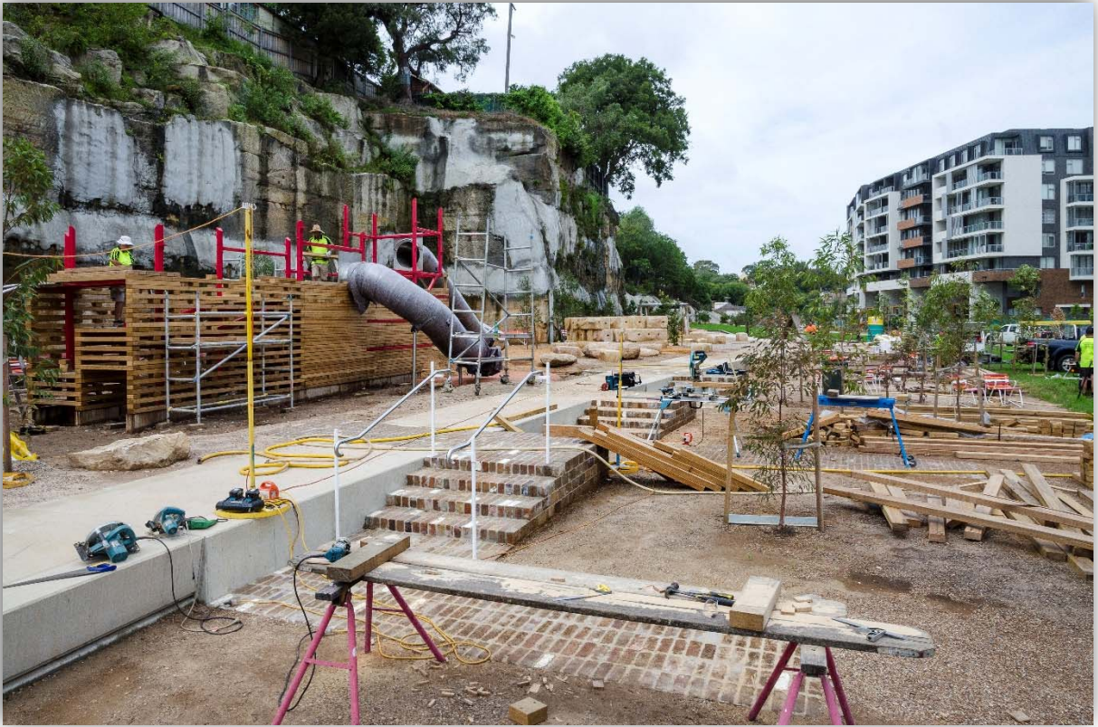
Location and Images of Harold Park (under construction May 2017)
